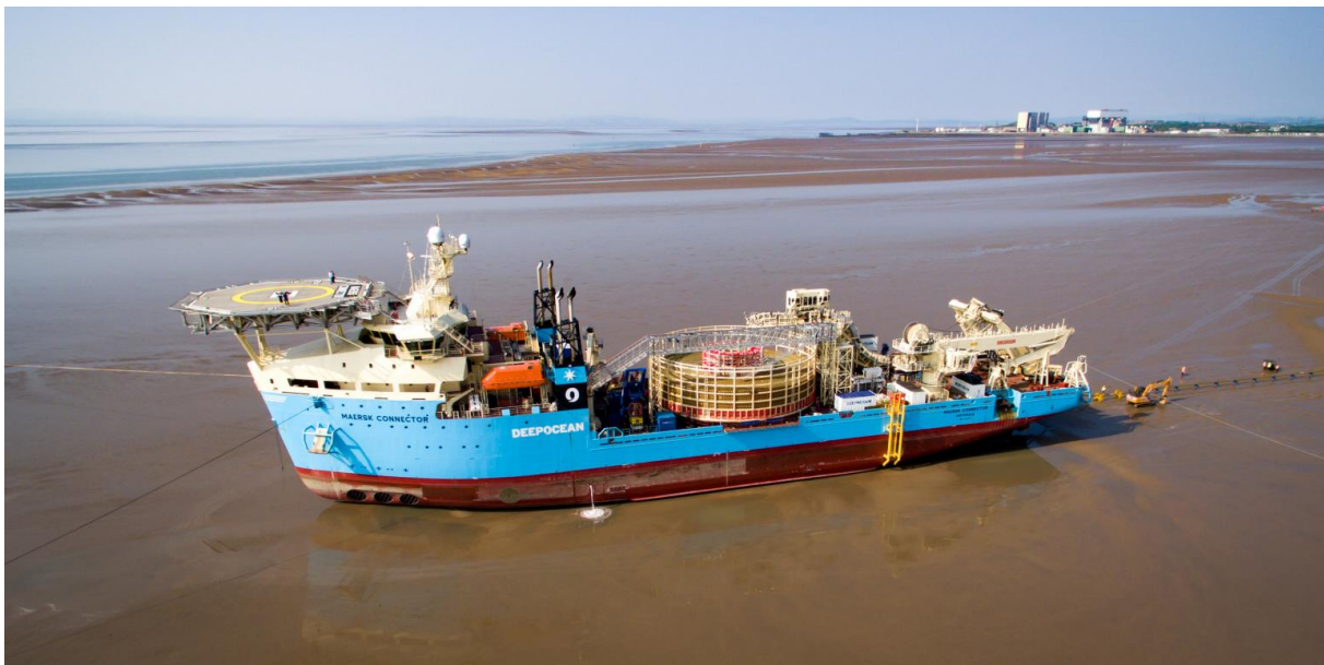
Figure 25: Delta Subsea's Connector performing a beached cable landing
